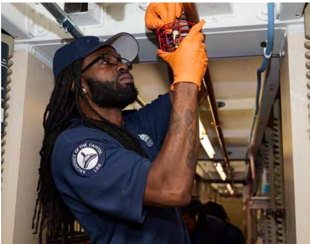
A plumber installs a cage around a newly fitted sprinkler head, part of the Library's Sprinkler System Replacement Project at the John Adams Building.
