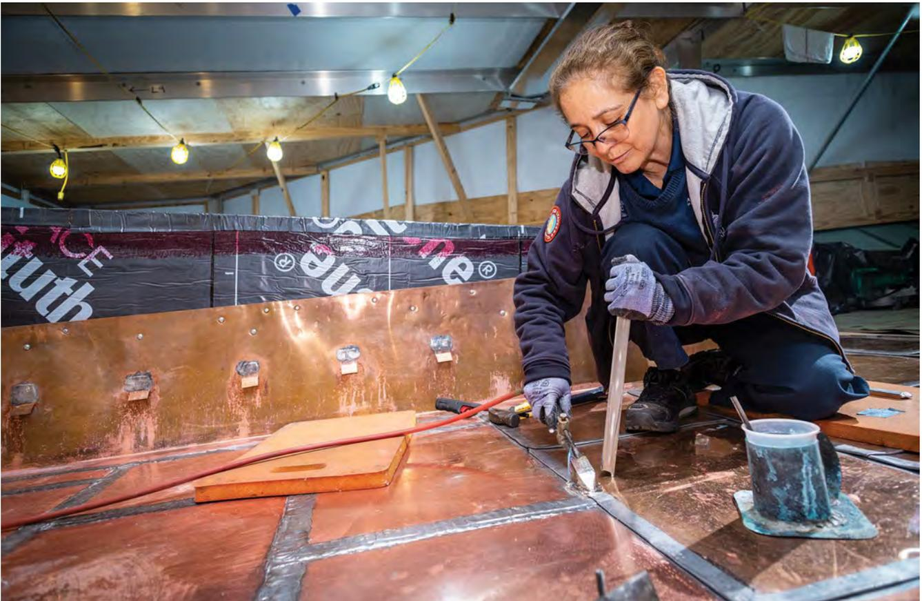
A professional from the AOC's Sheet Metal Shop installs new copper roofing near the Dome of the U.S. Capitol, ensuring durable protection for the historic structure.
