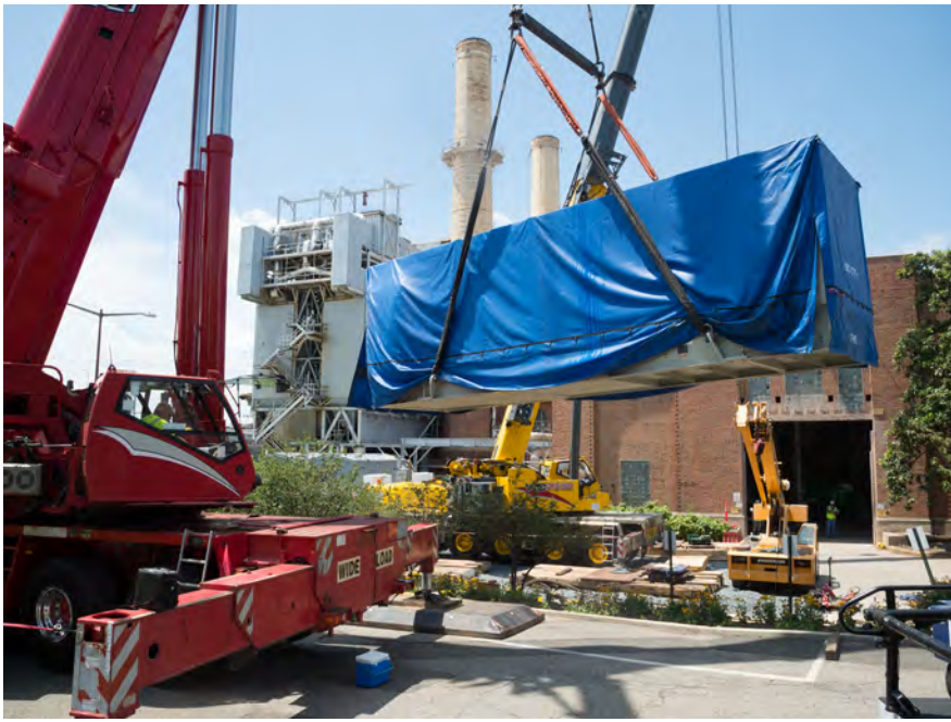
Left: From the biggest lifts .... Delivery of heat recovery steam generator and combustion turbine generator, part of Capitol Power Plant East Refrigeration Plant upgrades. Susanne Bledsoe, 7.24.2017 Right: To the subtlest brushstrokes .... Artist Robert Beckmann inpaints Citrus panel following installation. U.S. Botanic Garden Conservatory interpretive panels depicting the human cultivation of corn, cocoa, citrus, cotton, tea and rice were added to the permanent exhibit. Michael Dunn, 2.28.2005
