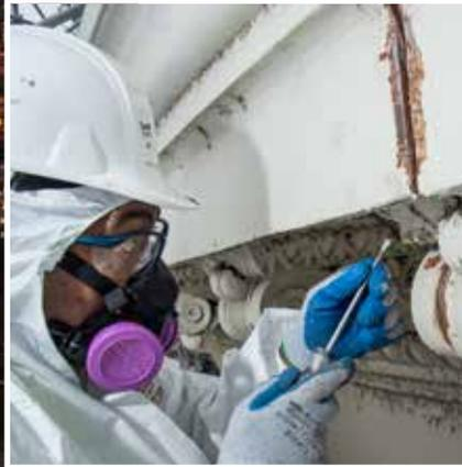
A worker removes sealant from the Dome.
