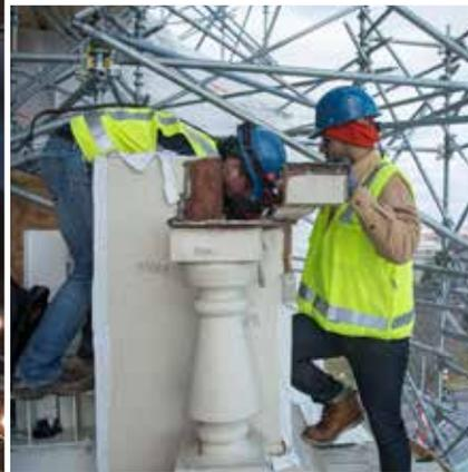
Workers disassemble the boiler plate balustrade.
