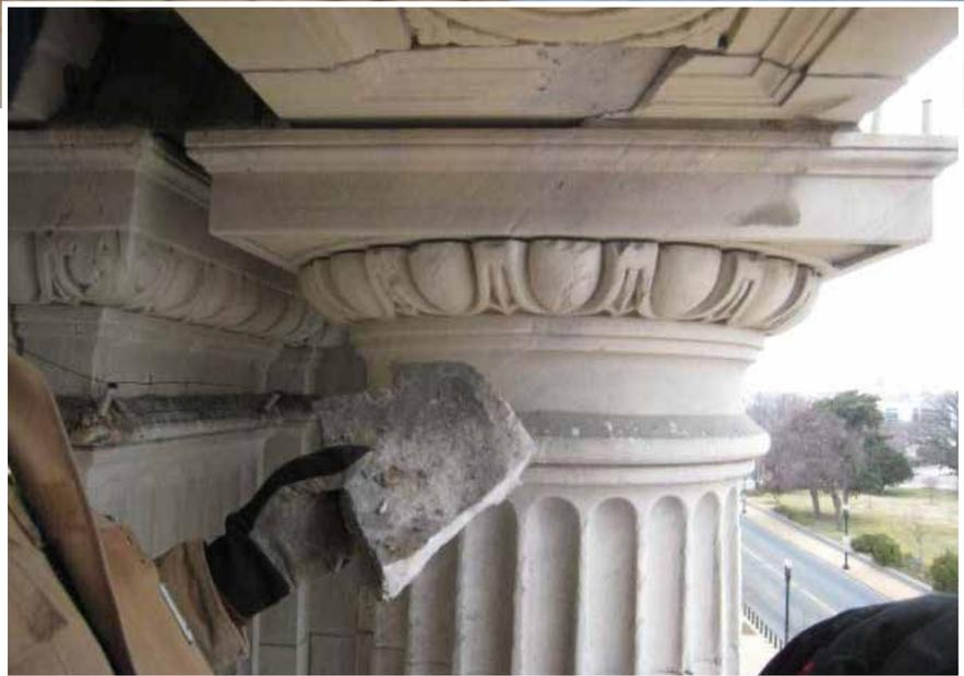
*Deteriorated stone from more than a century of weather damage and at left, an example of one of the many corroded pipes in the building.*
