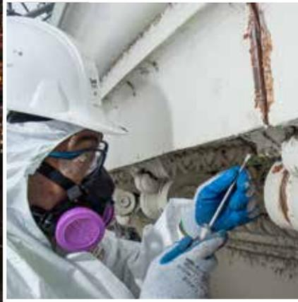
A worker removes sealant from the Dome.
