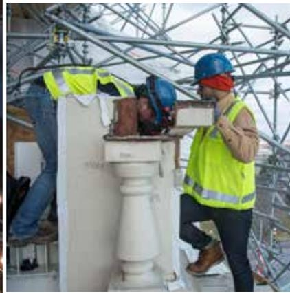
Workers disassemble the boiler plate balustrade.
